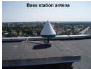
Fig. 7. Base station North (Kre)
